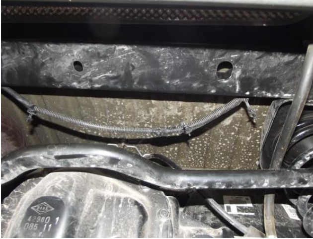
Photo 1 – Horizontal beam with wiring harness clips removed
